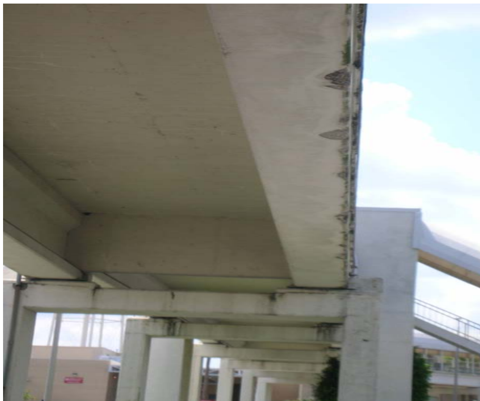
View of Skyway Underside
