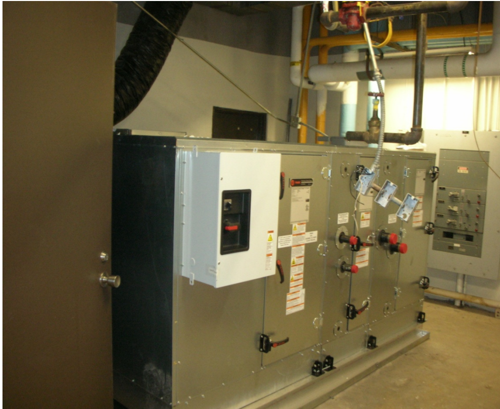
Picture Shows New AHU #16 in Place
