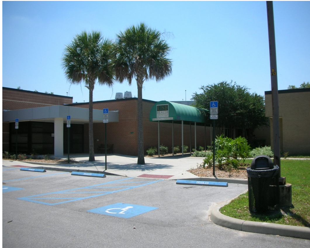
Picture MDT Lab Existing Entrance
