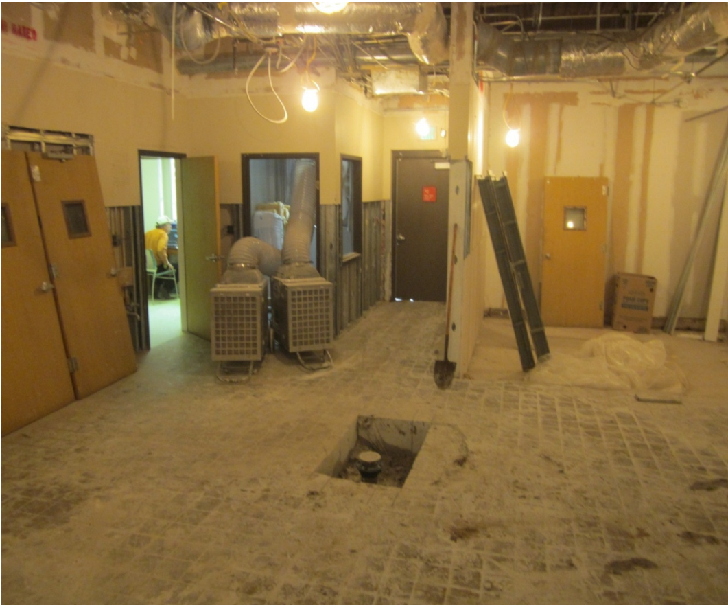
Picture MDT Lab Space Under Construction
