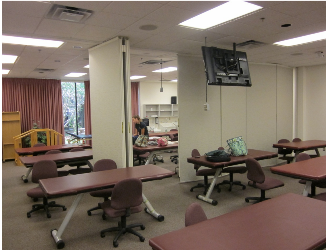
Picture of MDT 1010 Lecture Room Showing New Partition in Place
