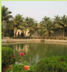
Settling pond that allows water from the Ganges River to settle before being treated for drinking
