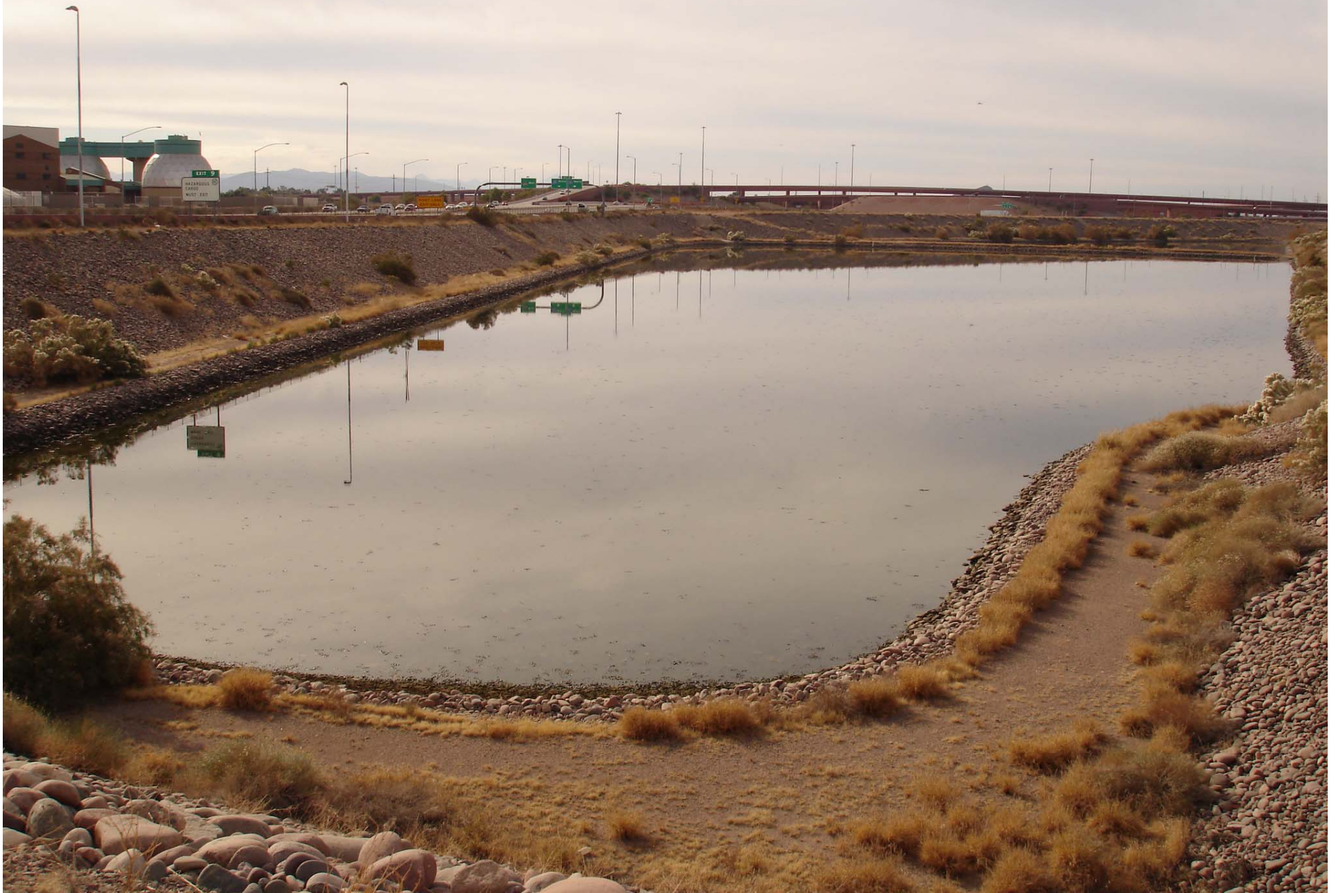
Infiltration pond for soil-aquifer treatment (SAT) in Mesa, Arizona.
