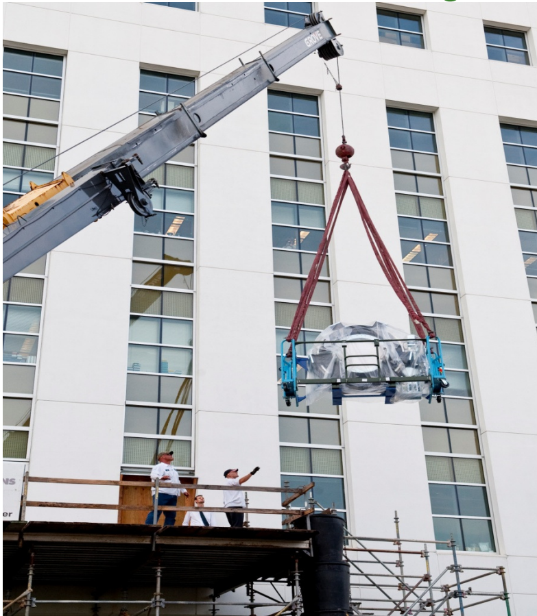
Picture Shows PET CT being lifted to 2 nd Floor
